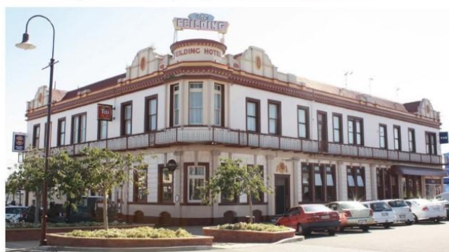
Feilding Hotel, 9 Manchester Square (constructed 1875-1910)
