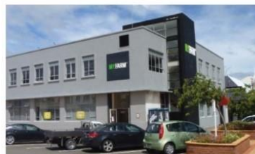
Photograph of 8 Manchester Street - (1949)
