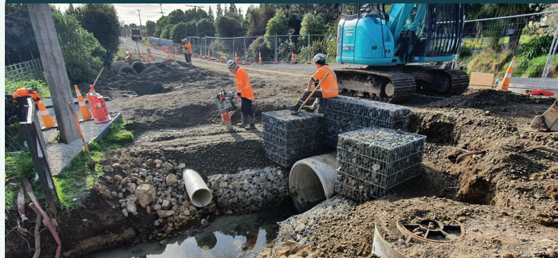
Stormwater upgrades Rongotea
