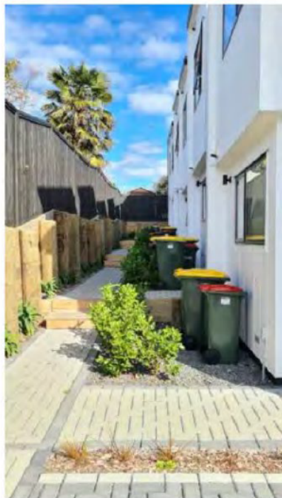
Figure 3: Bin storage needing stair access to get to the road frontage and not screened.
